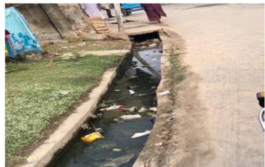
Figure 6. Poorly constructed roadside drains.
